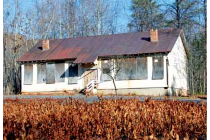
The Scrabble School in Rappahannock County, Va., shown here before restoration, now serves as senior citizens center.
