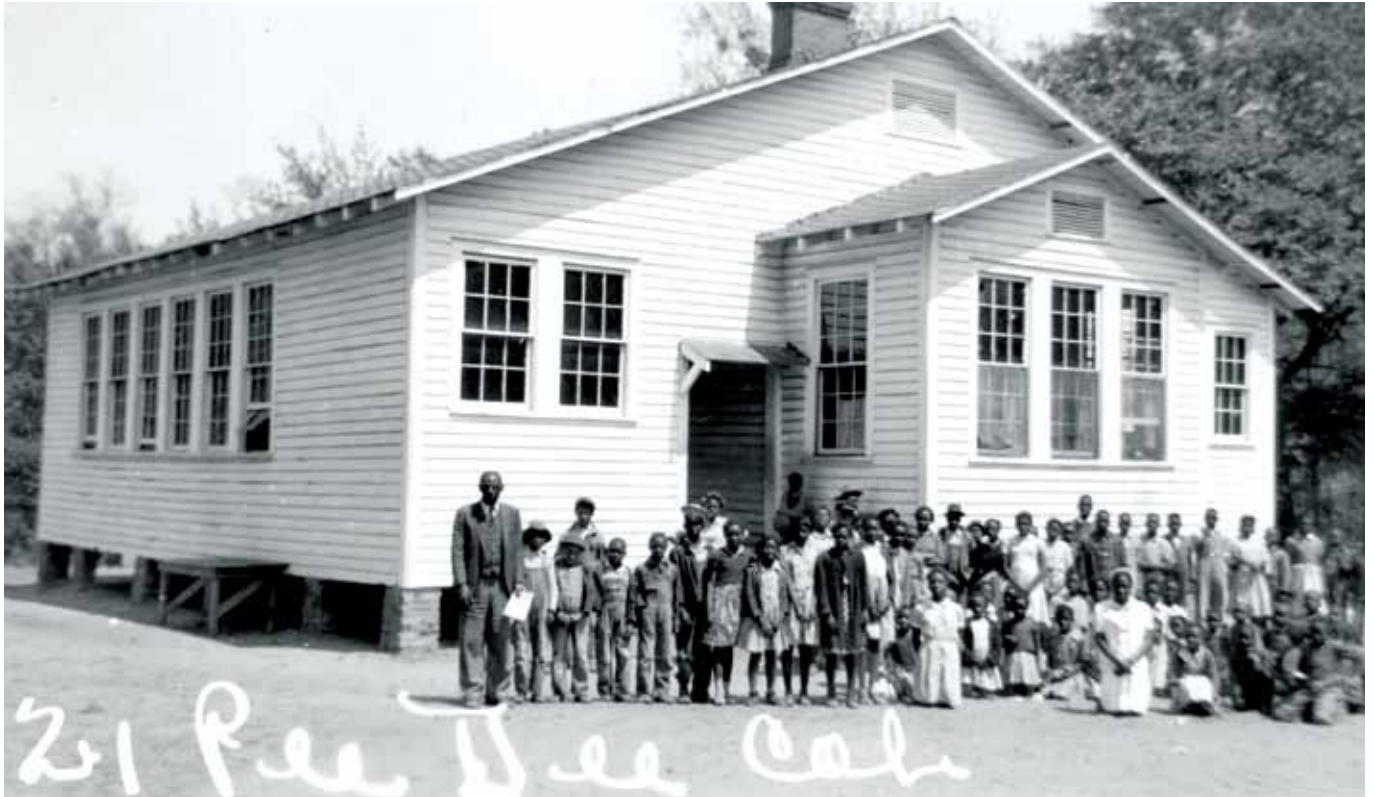
The Pee Dee Colored School in Marion County, S.C., a two-teacher school, was built in 1922-23. It followed Community School Plan No. 2-C, pictured on the opposite page. More two-teacher schools were constructed than any other type school.
